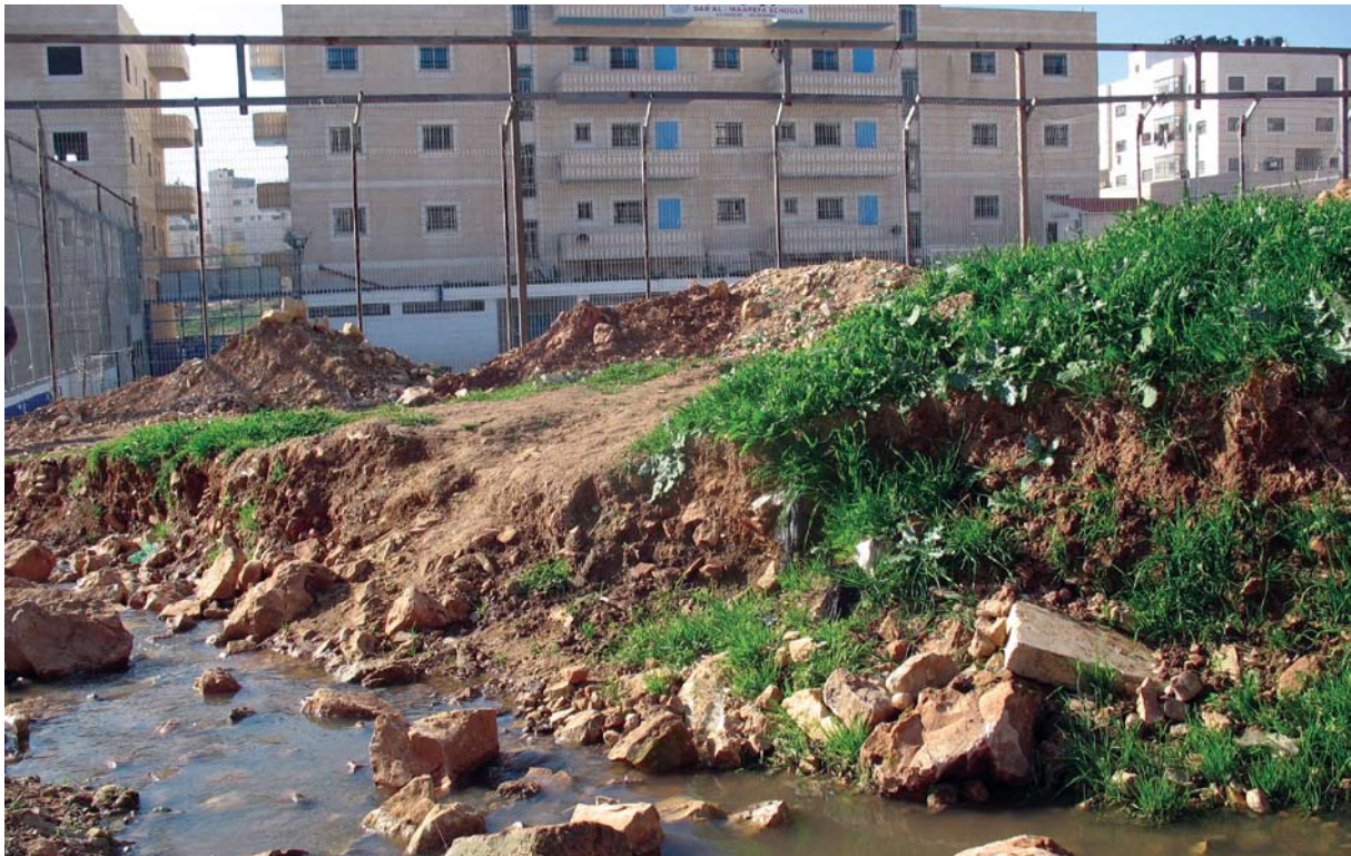
Sewage near a school in Kufr Aqab
